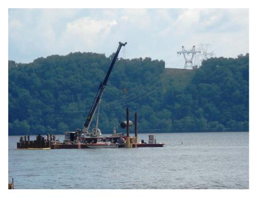
Figure 10, Wet Retrieval of MTBM
