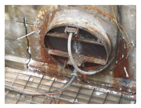
**Figure 9, Steel Casing Plug**
