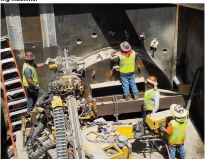
machine was able to work through the debris, the slurry discharge was problematic and there was concern that the MTBM would encounter mixed ground that could lead to a loss of face pressure and, in turn, result in serious ground control issues. Working beneath the rail lines added extra pressure.
