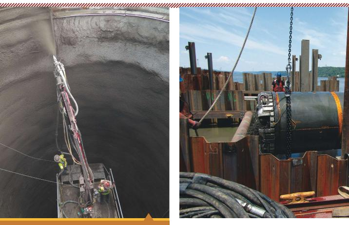
All shotcrete operations were preformed after all tunneling was completed from an elevated platform constructed by the contractor to support a shotcrete robot.
