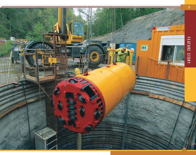
The project involved an 830-ft drive of 60-in. casing using a Herrenknecht AVN-1200 with rock cutterwheel.
