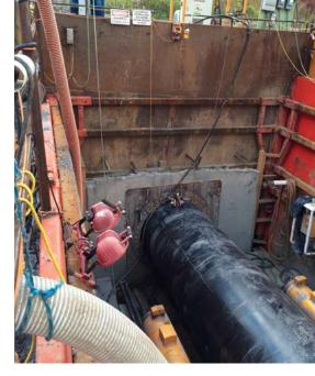
59-inch steel casing was used in lieu of 60-inch to increase overcut in self-supporting ground
