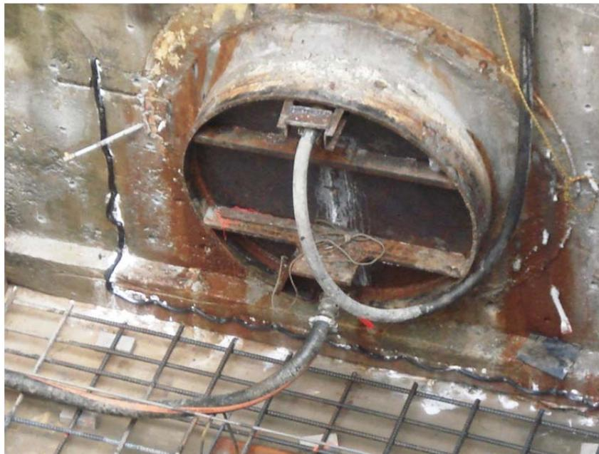
**Figure 9, Steel Casing Plug**
