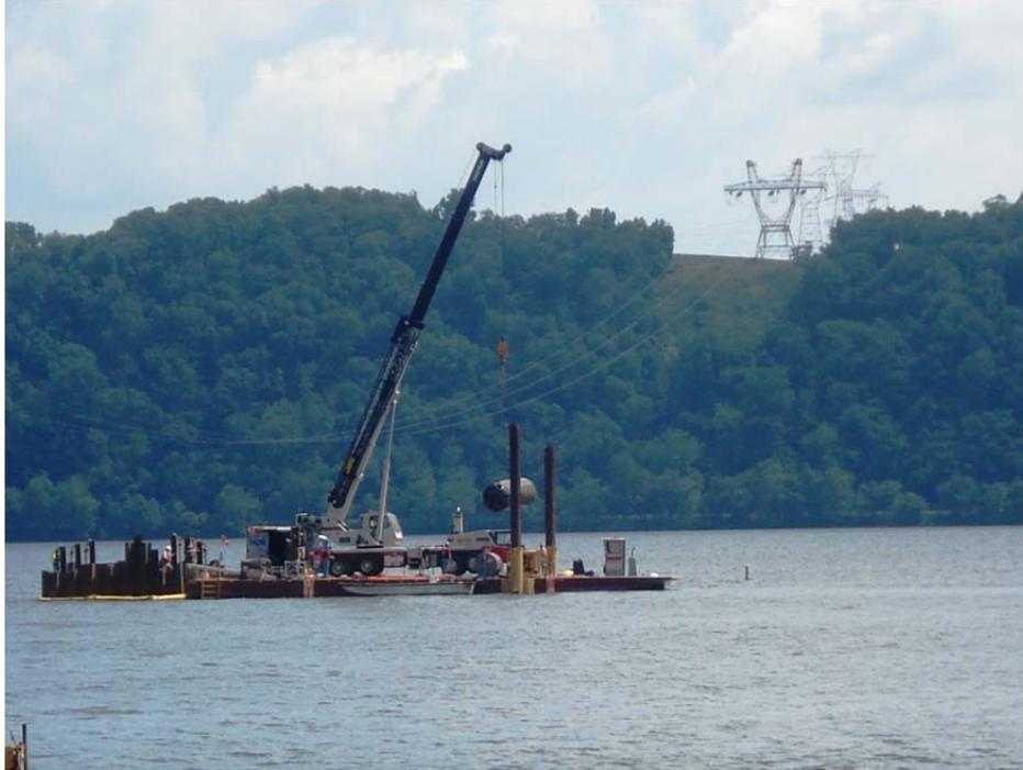
**Figure 10, Wet Retrieval of MTBM**
