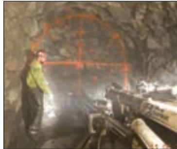
The tunnel line and grade and tunnel cross-sections were to be surveyed at maximum 20ft stations. Tunnel cross-sections were to be plotted and submitted to the engineer verifying excavation clearances throughout the tunnel before starting the application of any final lining.
