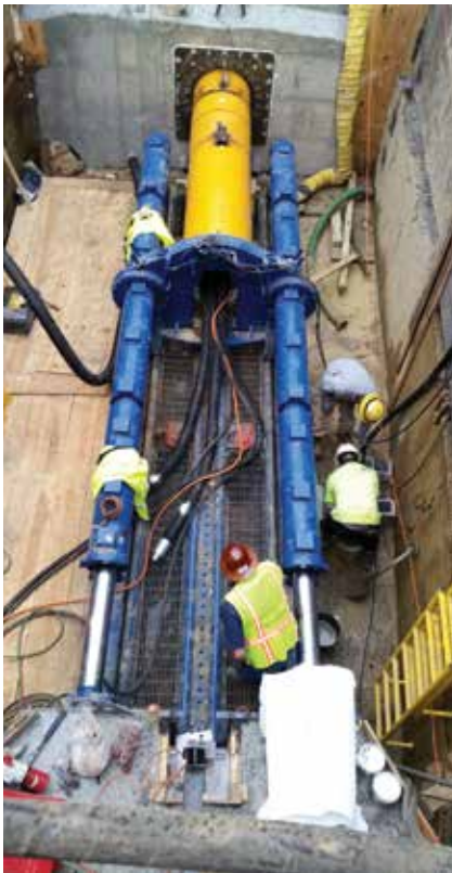
MTBM launch @ College Drive Waterline Project
