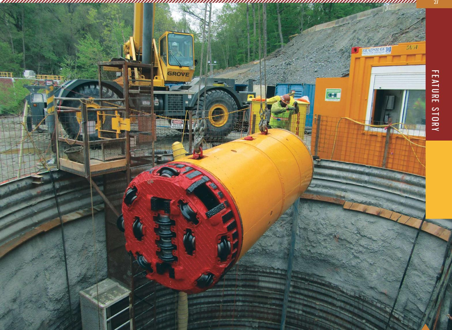
The project involved an 830-ft drive of 60-in. casing using a Herrenknecht AVN-1200 with rock cutterwheel.
