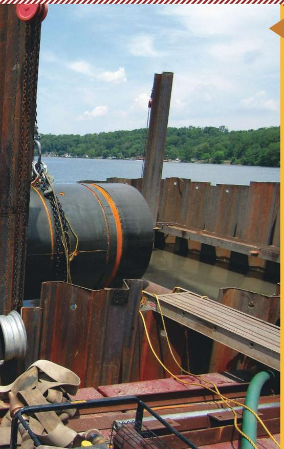
rine open-cut construction. Spatial constraints within the shaft prohibited the parallel bores, and based on Bradshaw's previous project experience, it proposed one 60-in. steel casing tunnel be installed from the wet well shaft 830 ft to the intake location.
